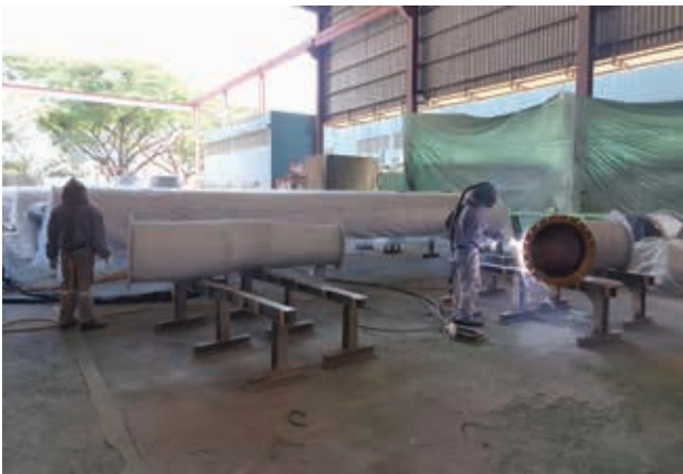
Figure 4: Corrosion Prevention – Application process
