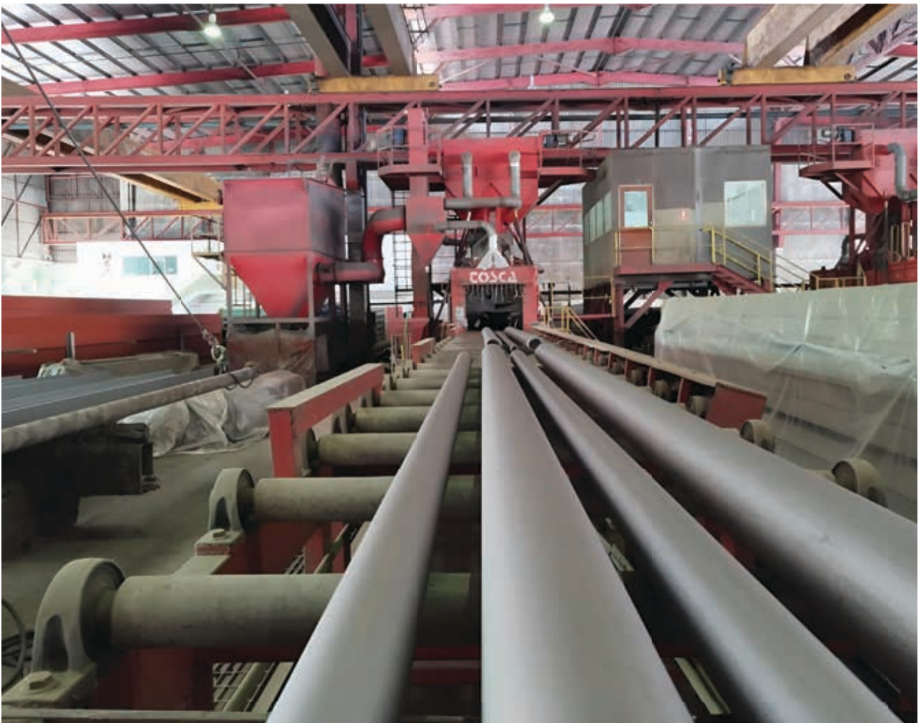
Figure 3: Corrosion Prevention – Piping works
